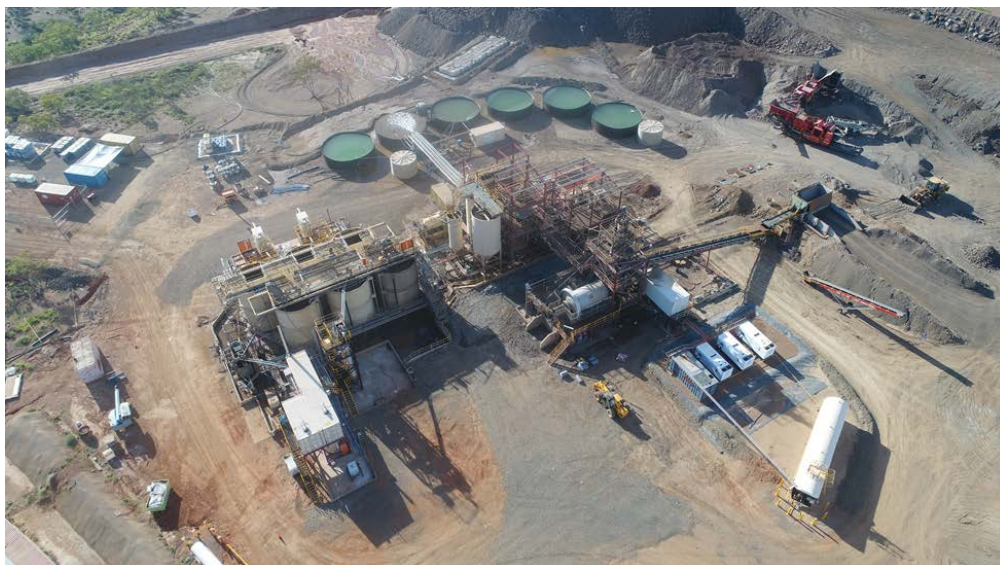
Aerial View of Lorena Processing Plant
