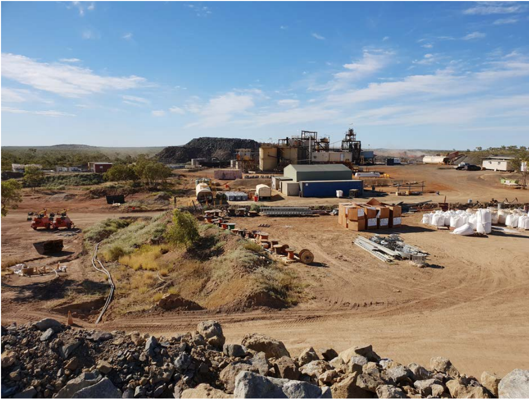
ROM stockpile in background behind processing plant – photo taken from tailings dam wall
