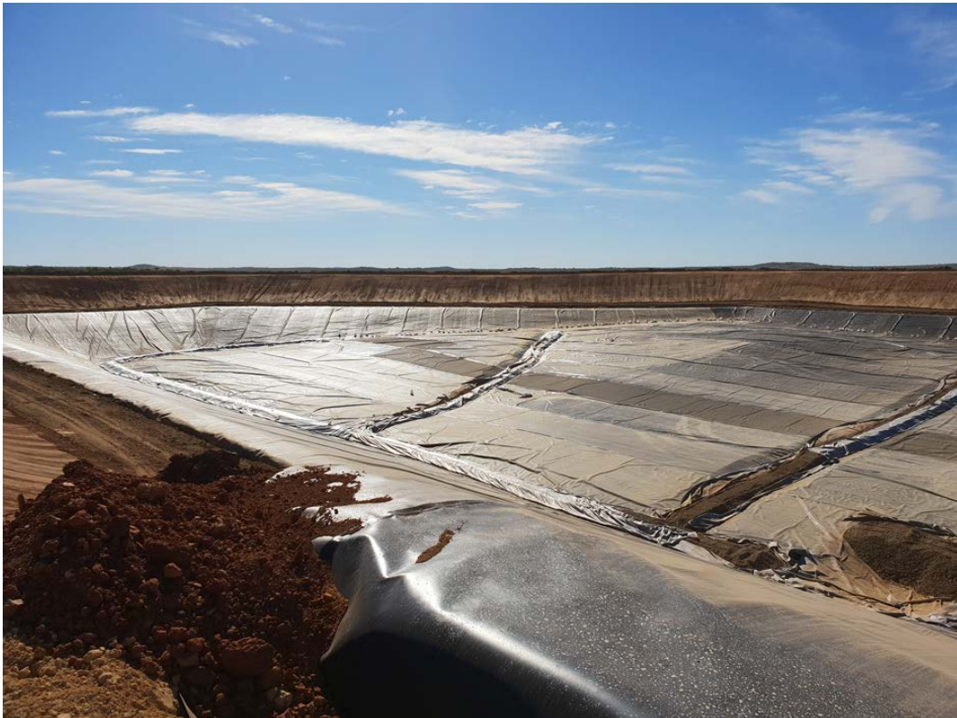
Second cell of the Lorena tailings dam liner being installed.
