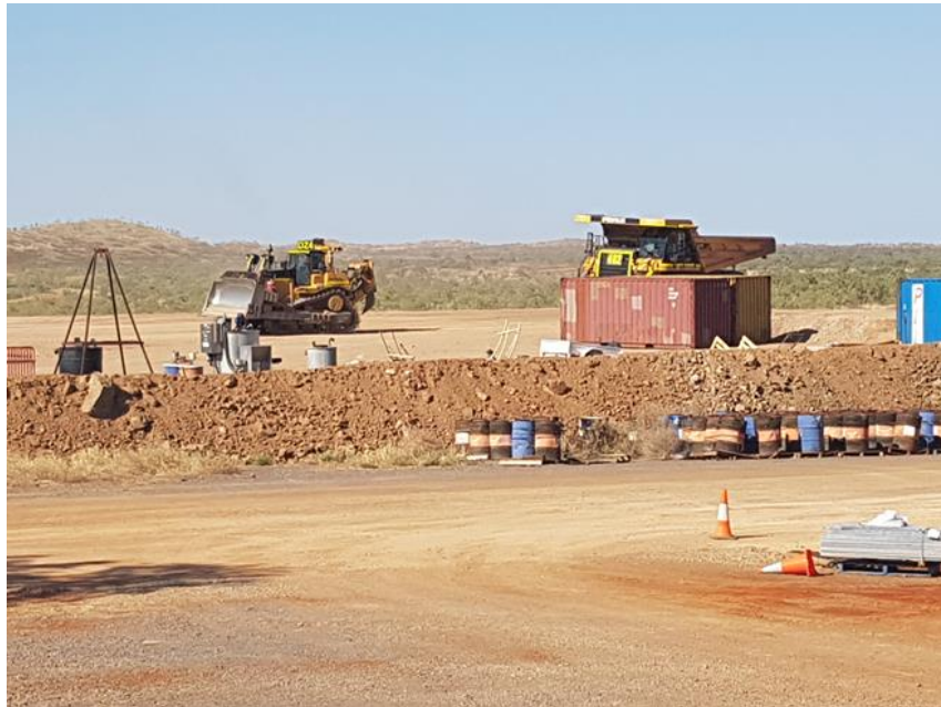
Construction of the tailings dam
