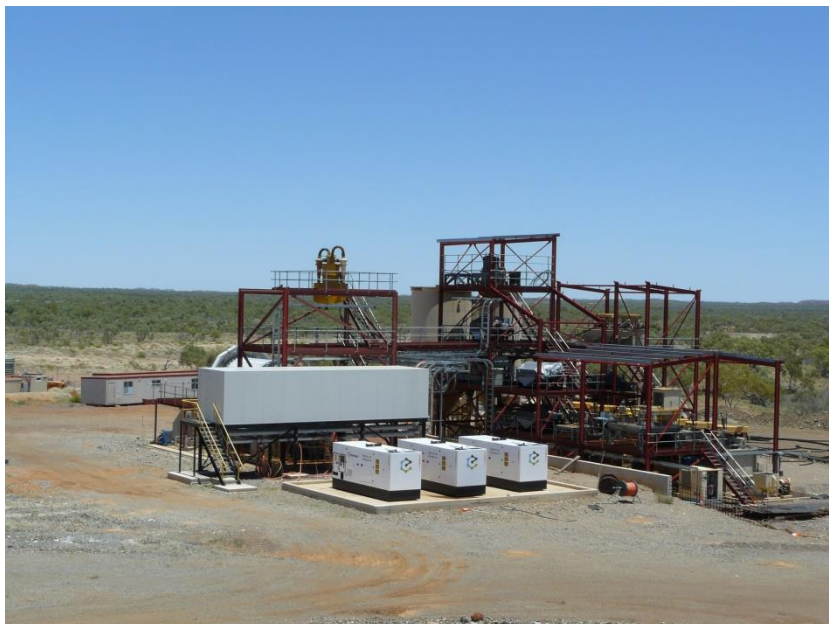
Lorena Concentrator Plant
