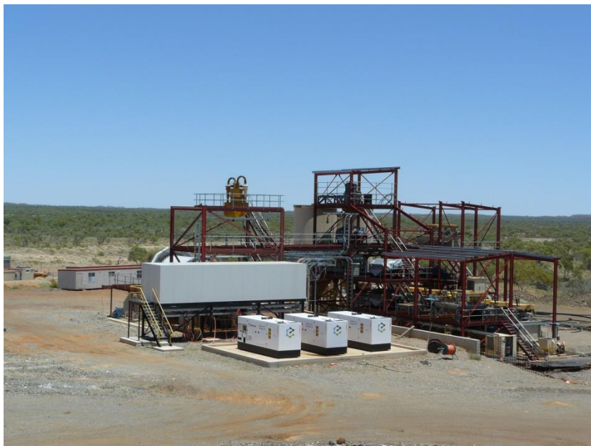
Lorena Concentrator Plant
