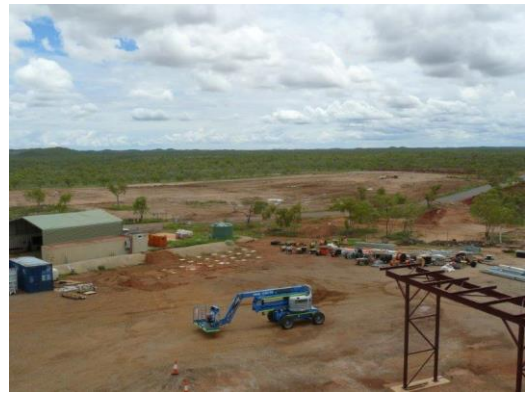
Tailings dam area grubbed in background
