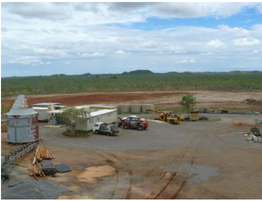
Preparation of waste rock dump in background
