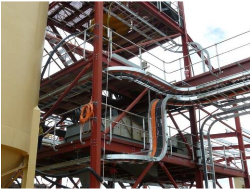
Electrical cabling in progress
